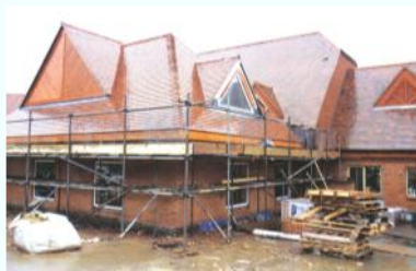
Building work underway 1990
